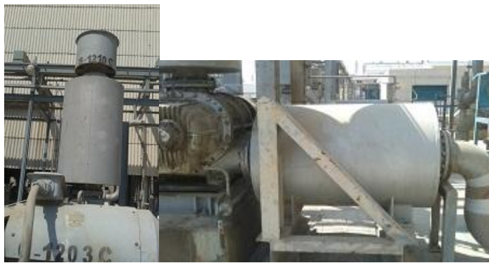
FABRICATED SAMPLE IN THE SITE
